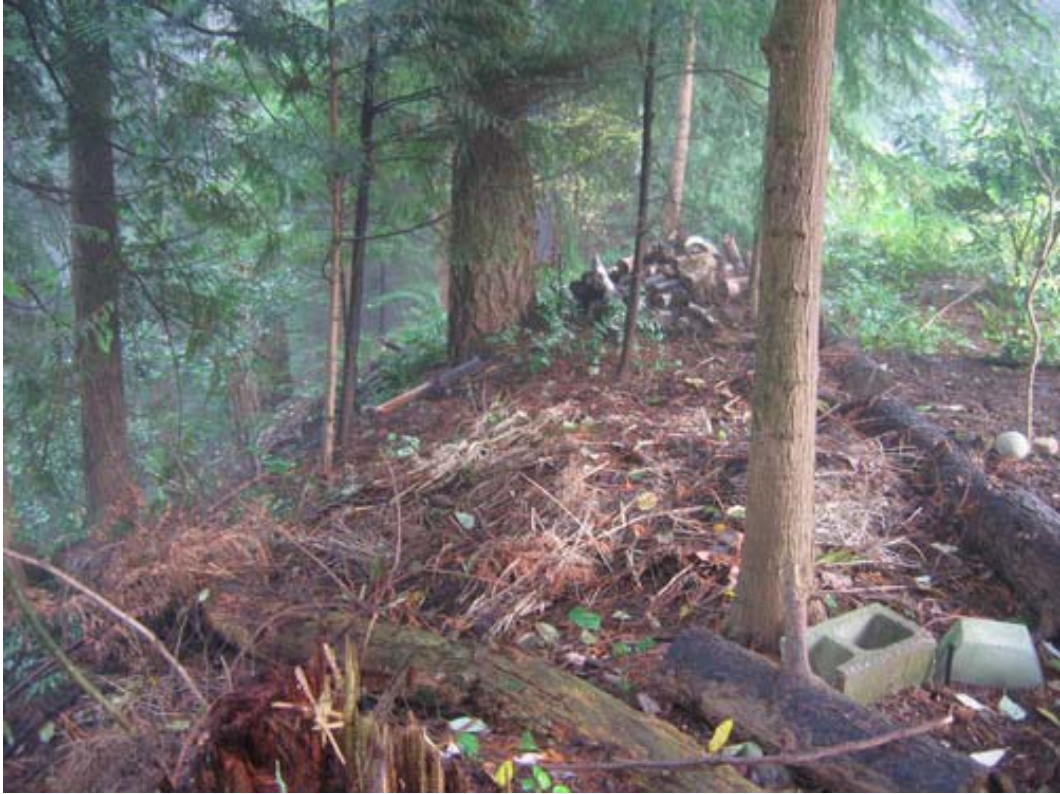
Figure 3. 2386 Carman Place – View looking east along crest
