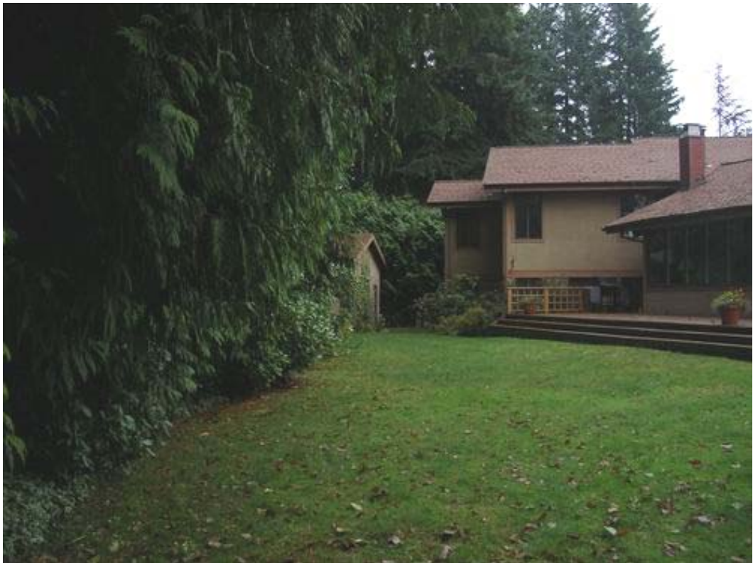
Figure 2. 2372 Carman Place – View along crest line towards the house
