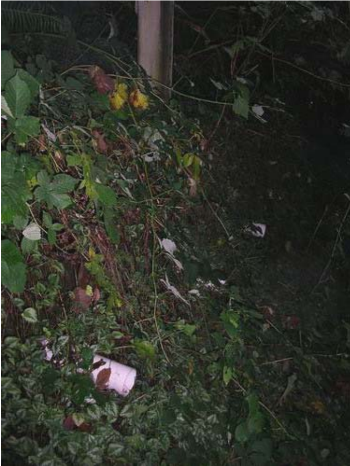
Figure 3. 2360 Carman Place – Drainage pipe exit on slope
