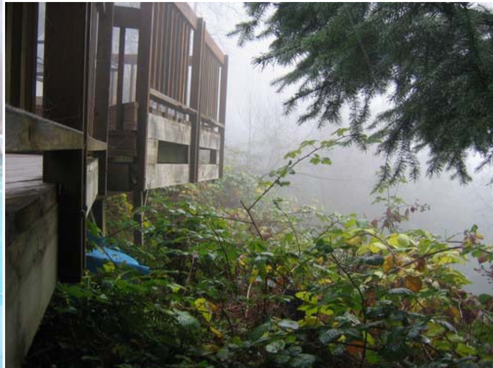
Figure 4. 2379 Carman Place – View looking SE along crest
