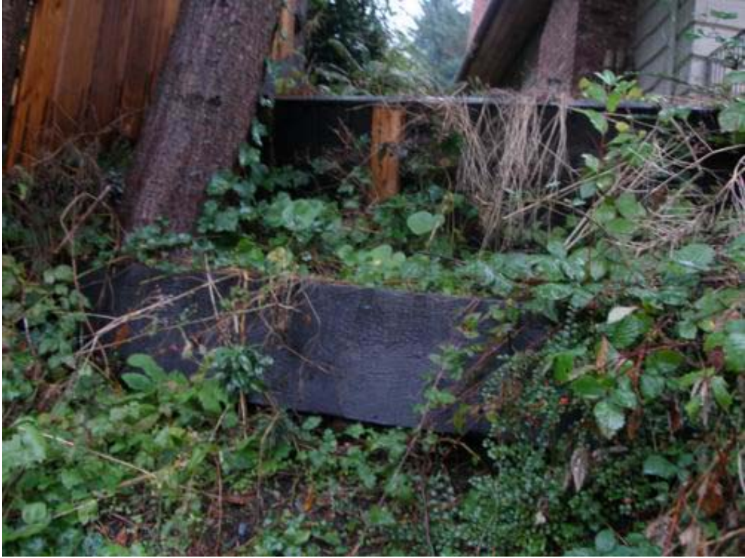
Figure 3. 2391 Carman Place – Timber retaining wall
