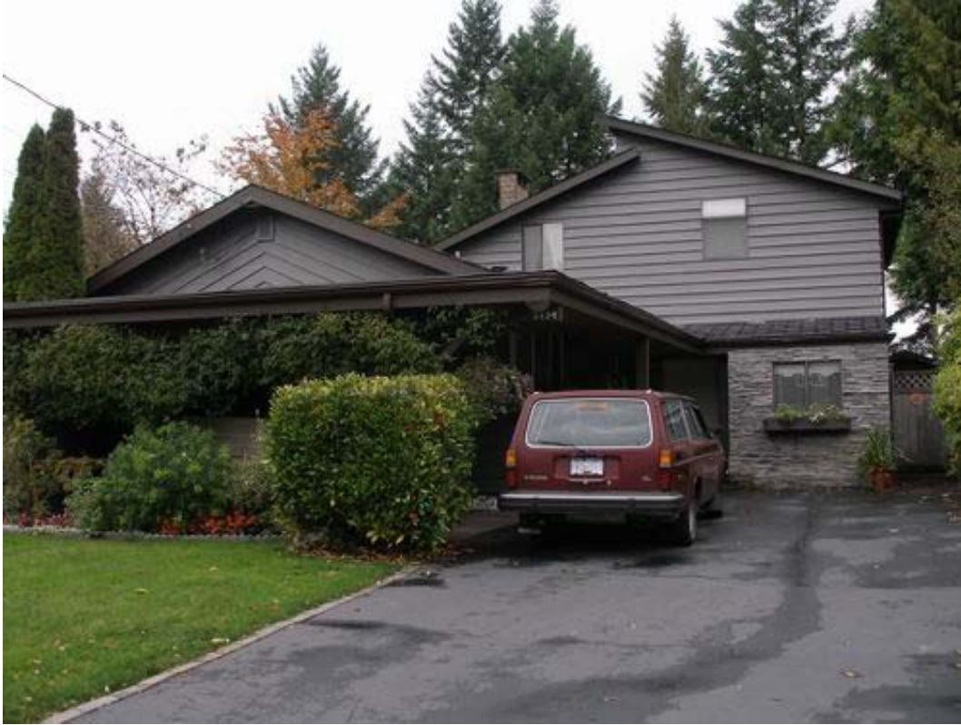
Figure 1. 2454 Hayseed Close – Front of the house
