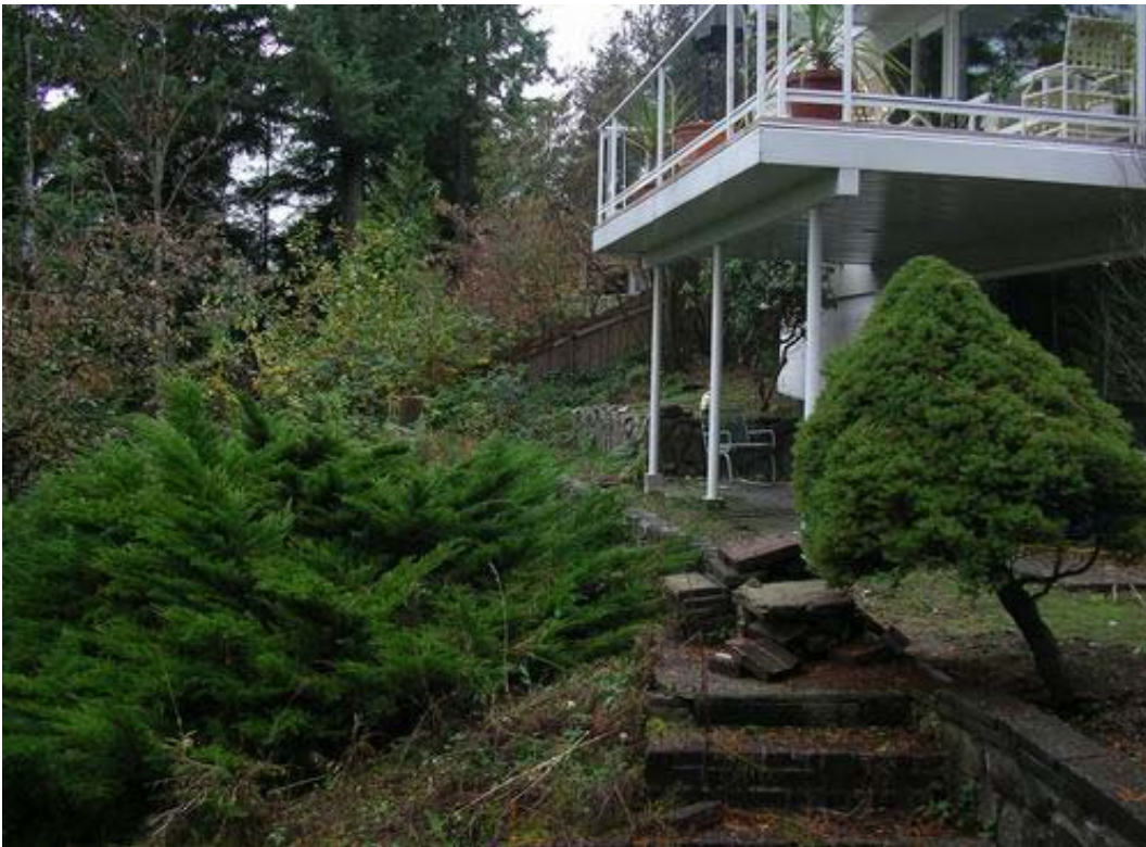
Figure 2. 2462 Hayseed Close – View of backyard looking north
