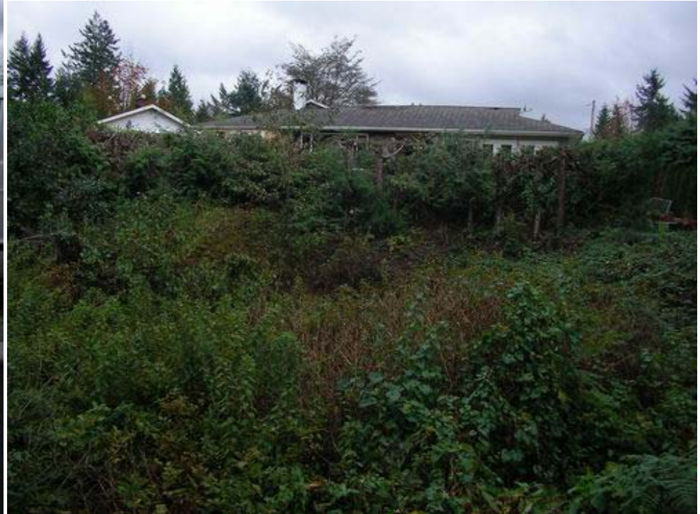
Figure 2. Hayseed-Layton Gully – View of 2442 Hayseed looking north from south side of gravel pit
