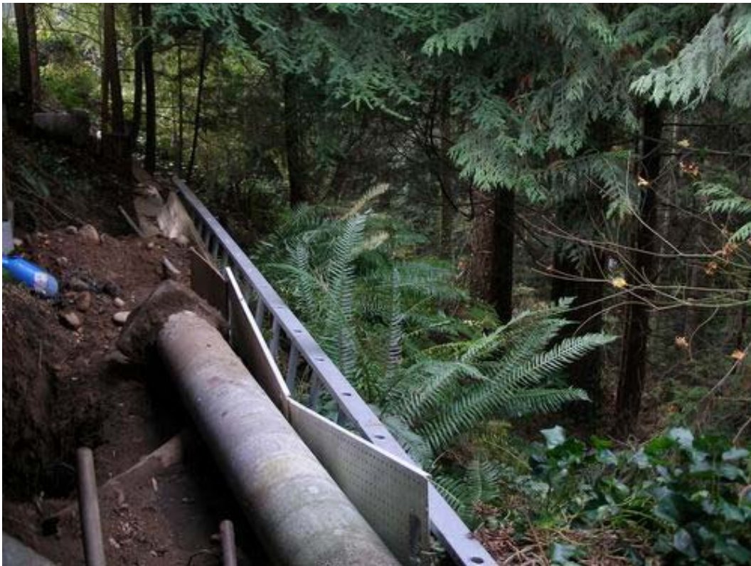
Figure 4. 2474 Hayseed Close – In-progress renovation of deck supports
