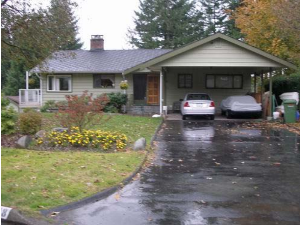
Figure 1. 2448 Hayseed Close – Front of the house
