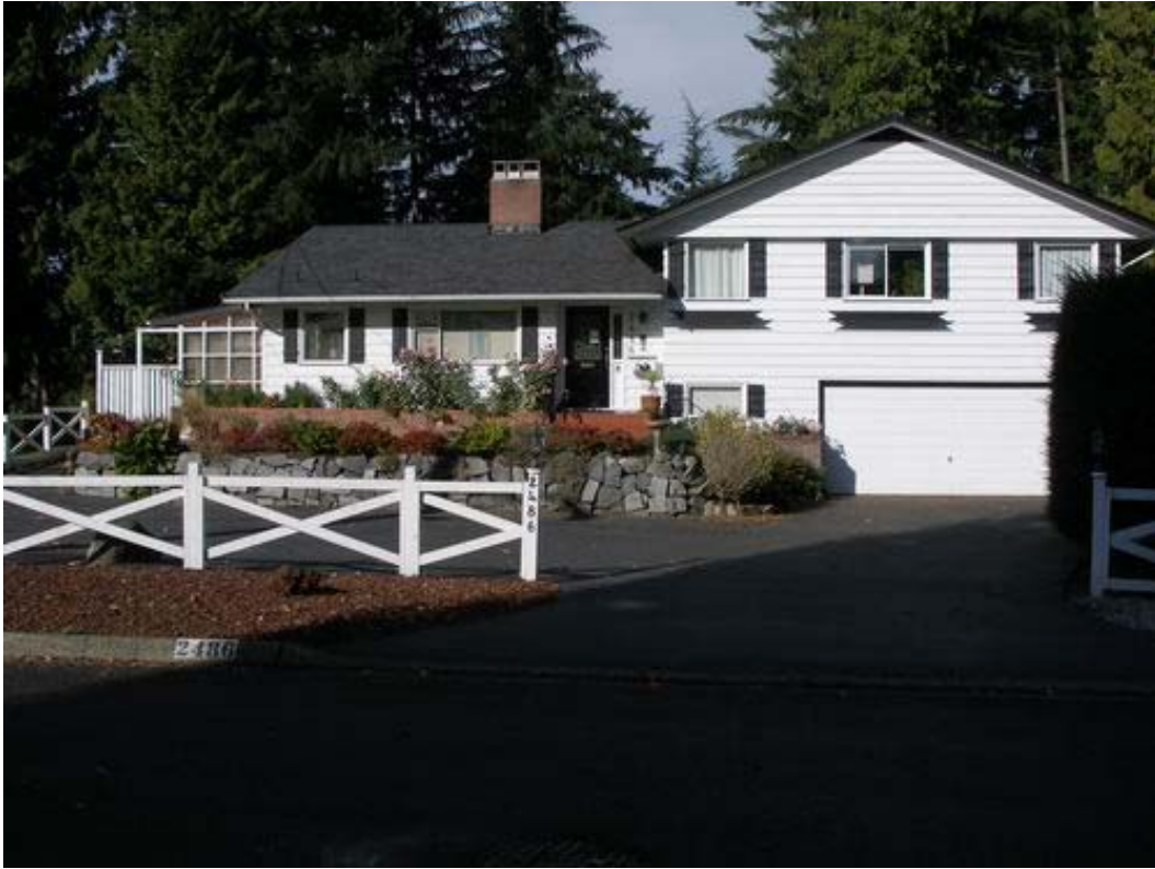
Figure 1. 2486 Hayseed Close – Front of the house
