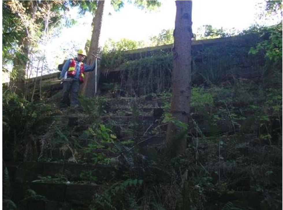
Figure 4. 2480 Hayseed Close – Timber crib retaining wall
