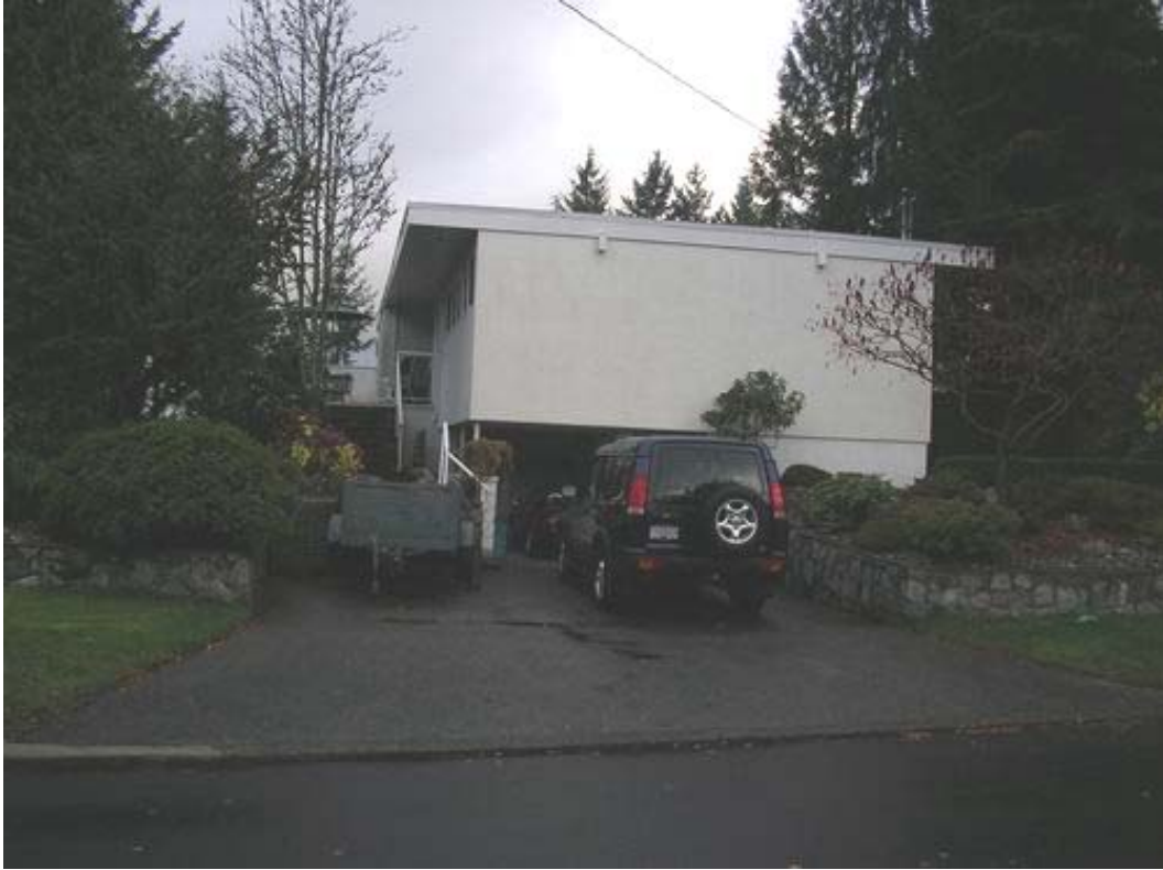
Figure 1. 2462 Hayseed Close - Front of the house
