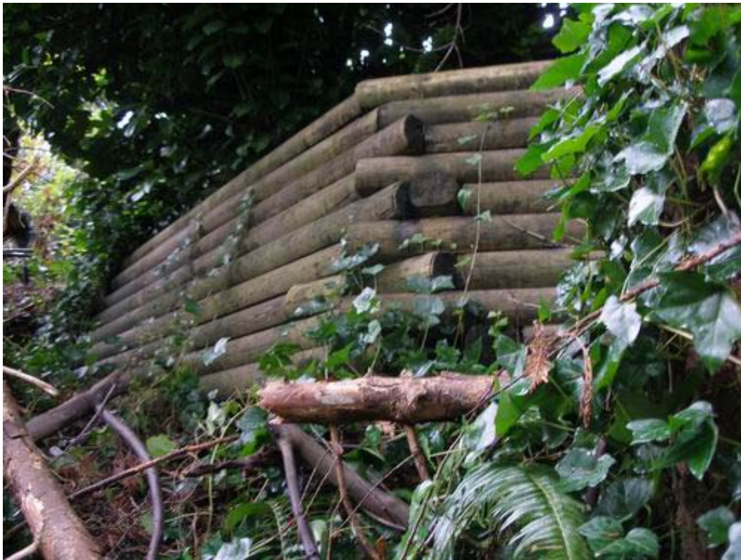
Figure 2. 2454 Hayseed Close – Timber crib retaining wall
