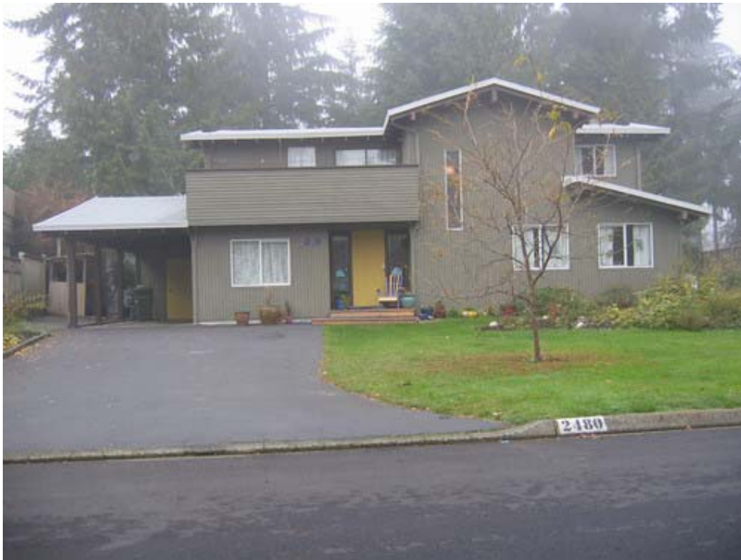
Figure 1. 2480 Hayseed Close – View of front of house
