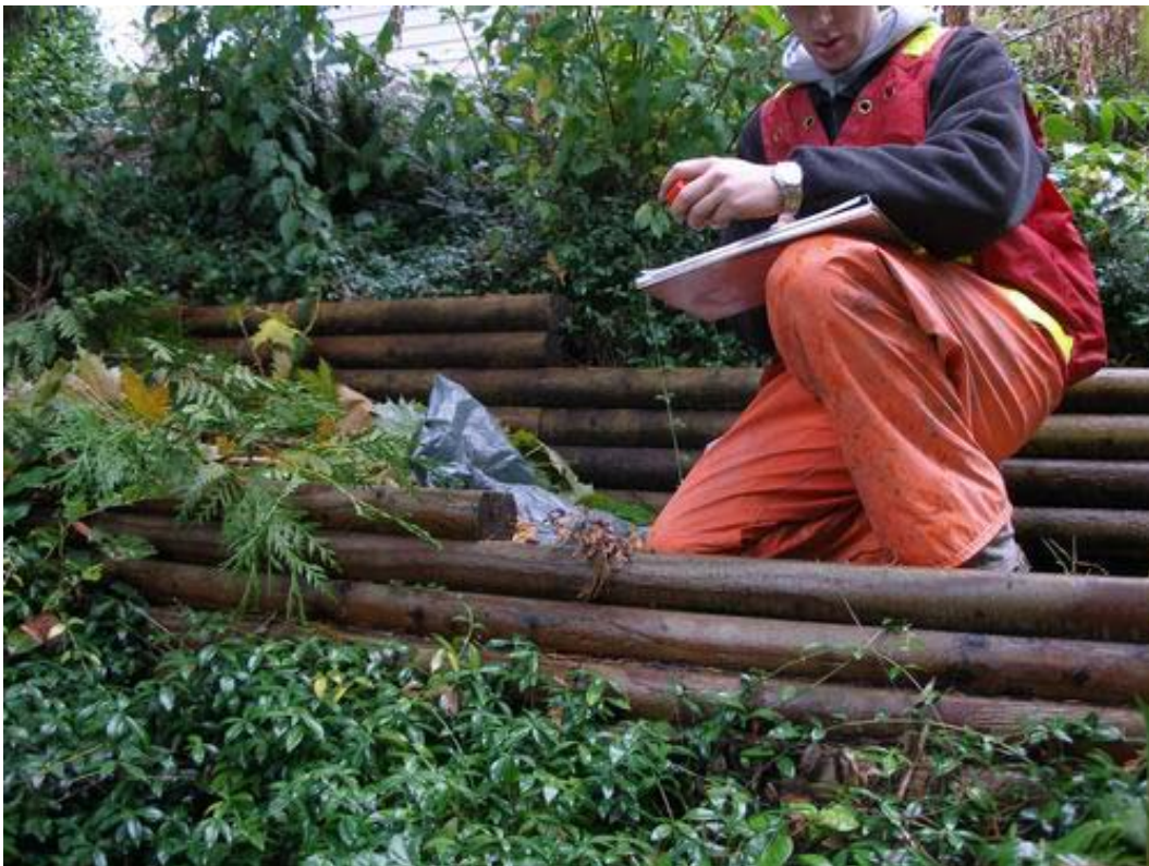
Figure 2. 2448 Hayseed Close – Timber crib retaining structure
