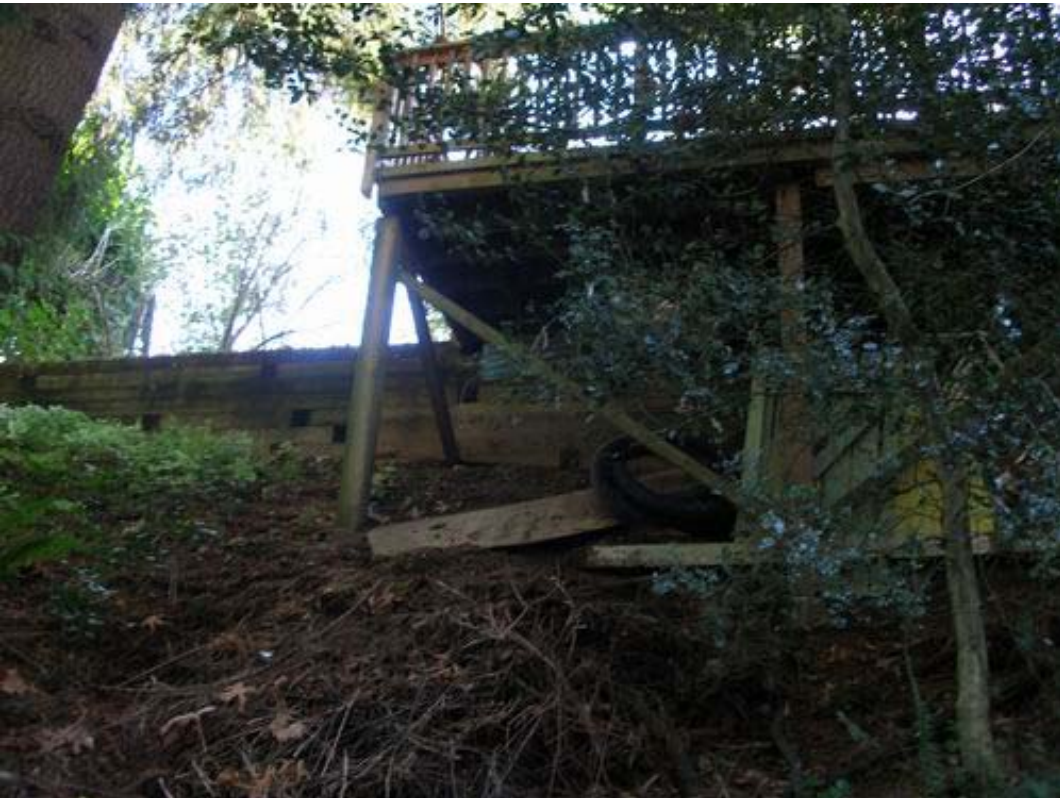
Figure 2. 2141 Berkley Avenue - Timber crib retaining wall
