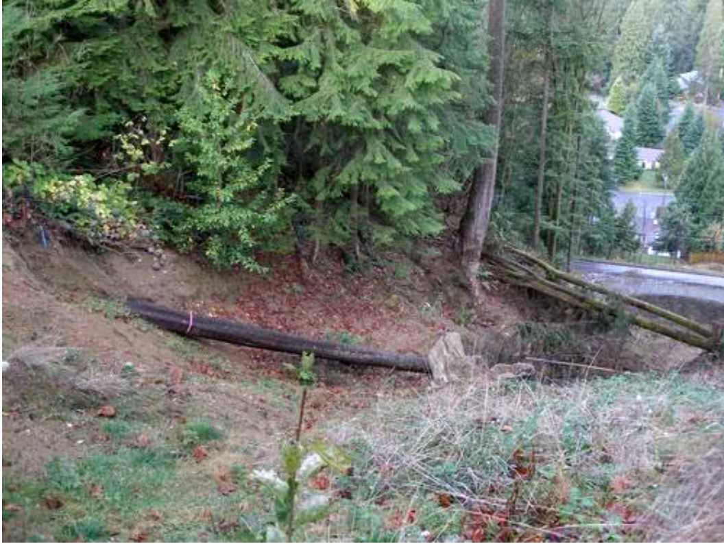
Figure 3. 2175 Berkley Avenue – View down-slope of January 2005 slide
