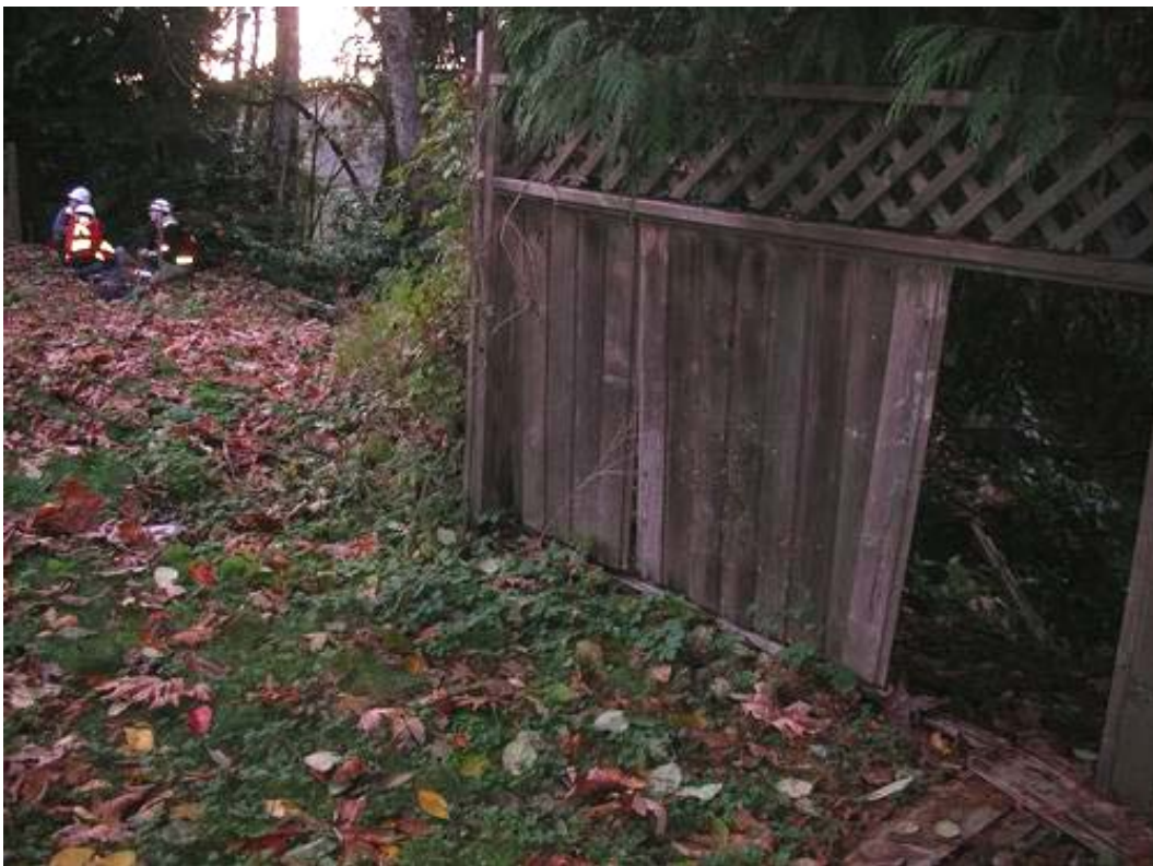
Figure 2. 2205 Berkley Avenue – View along crest of slope
