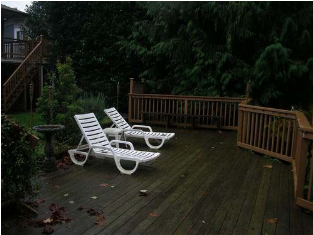
Figure 4. 2217 Berkley Avenue – View of backyard looking south
