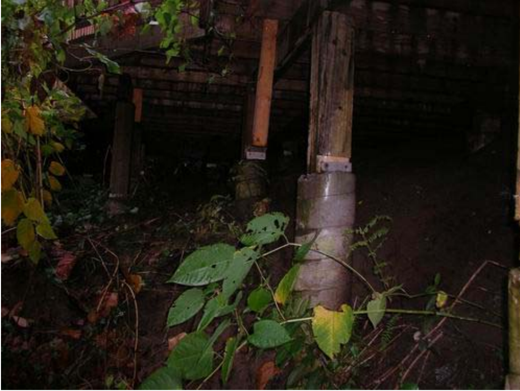
Figure 3. 2217 Berkley Avenue – Deck supports
