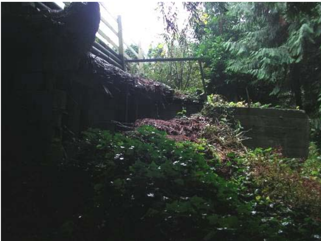
Figure 4. 2265 Berkley Avenue – Concrete retaining wall
