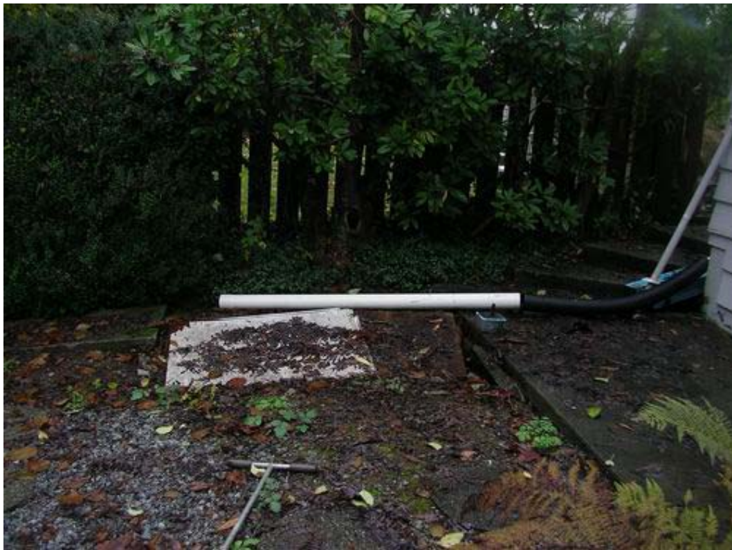
Figure 4. 2249 Berkley Avenue – Drainage pipe exit
