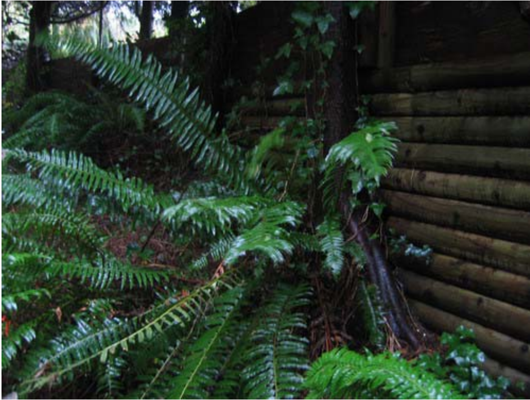
Figure 5. 2279 Berkley Avenue – Timber crib retaining wall
