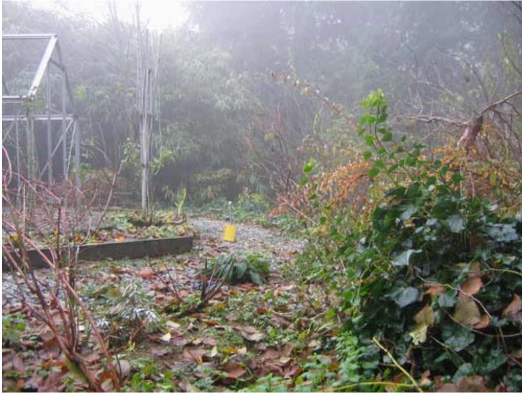
Figure 3. 2249 Berkley Avenue – View looking south along crest with marked piezometer
