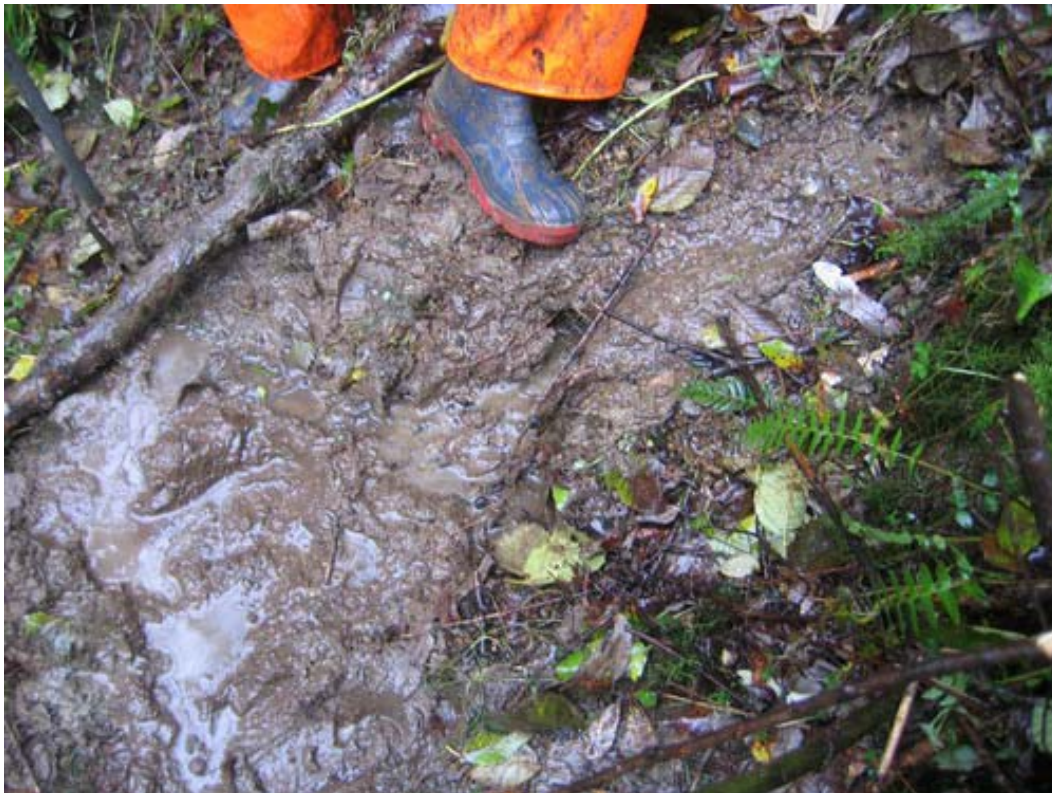
Figure 2. 2391 Berkley Avenue – Ponding of water from seepage
