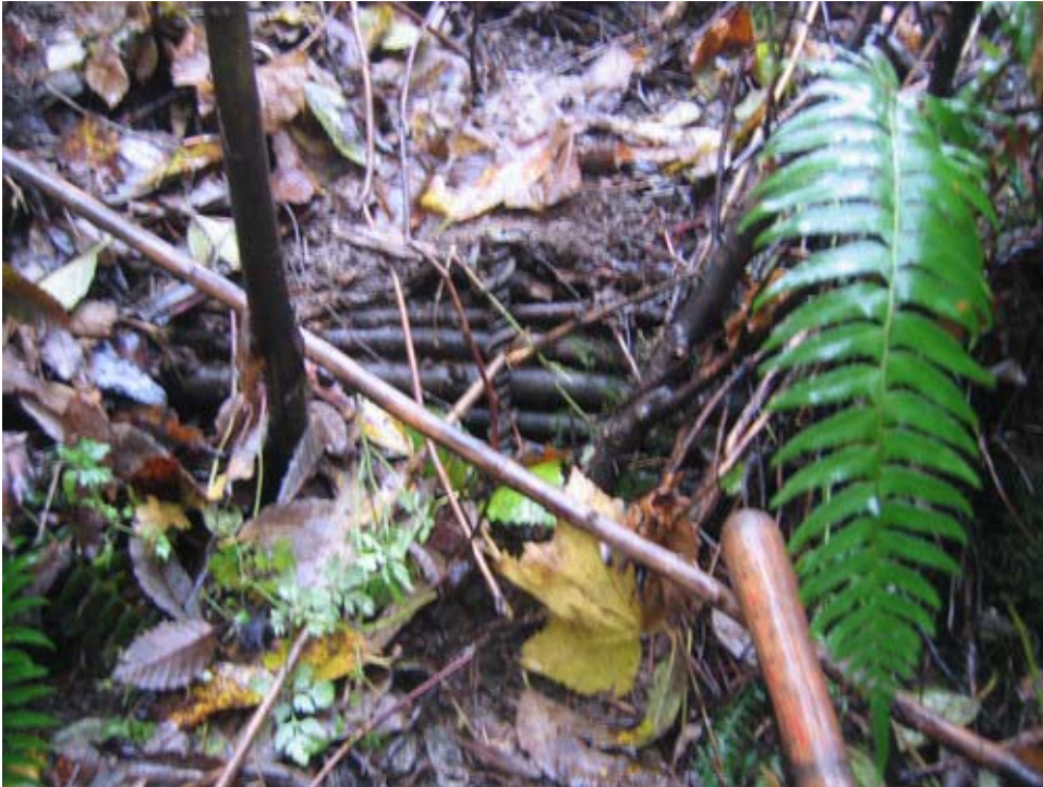
Figure 3. 2391 Berkley Avenue – Close up of rebar and stick retaining structure
