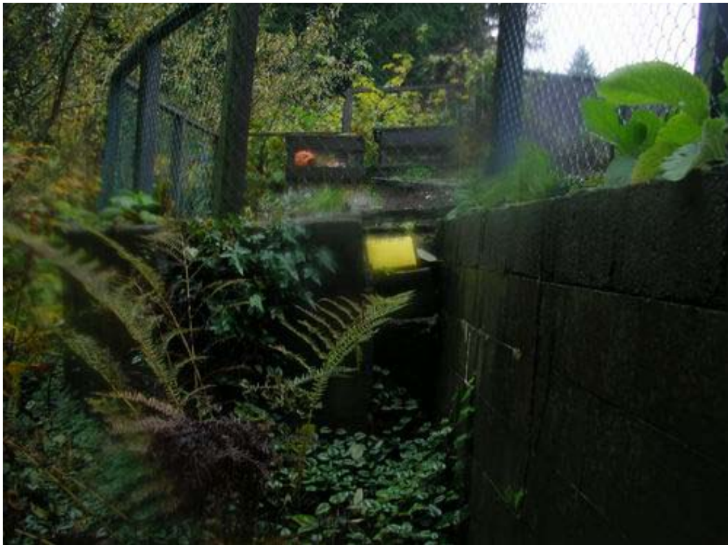
Figure 4. 2377 Berkley Avenue – Concrete retaining wall
