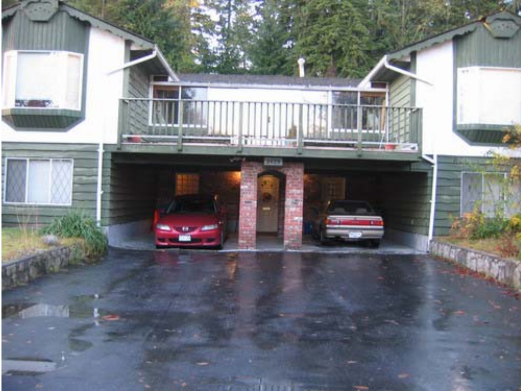
Figure 1. 2425 Berkley Avenue – Front of the house
