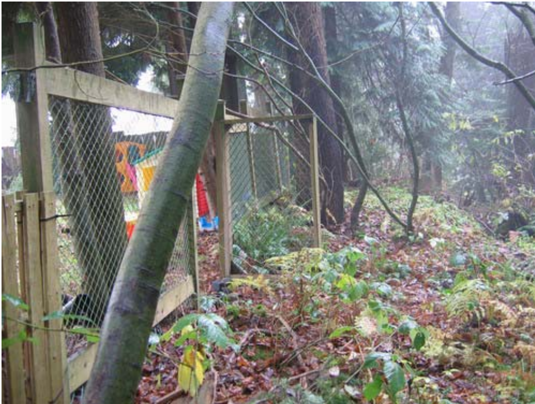
Figure 2. 2425 Berkley Avenue – View looking south along fence
