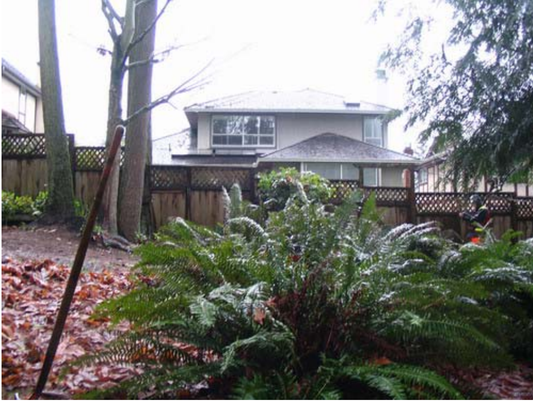
Figure 1. 2433 Mowat Place - View of house from crest
