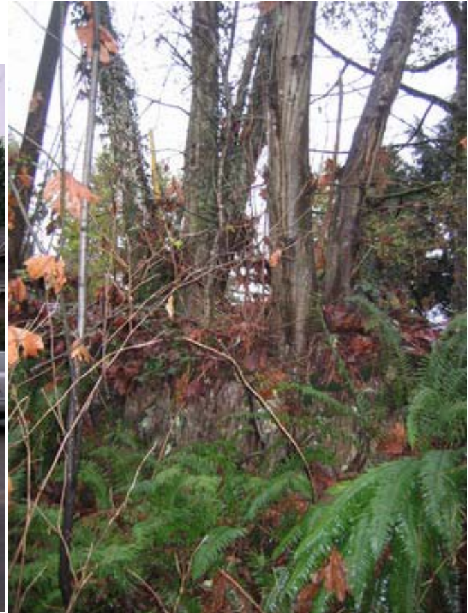
Figure 2. 2429 Mowat - Eroded root system of tree near crest
