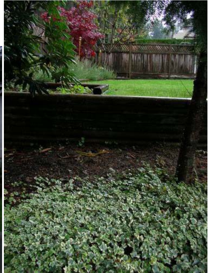
Figure 2. 2437 Mowat Place – View from crest to retaining wall
