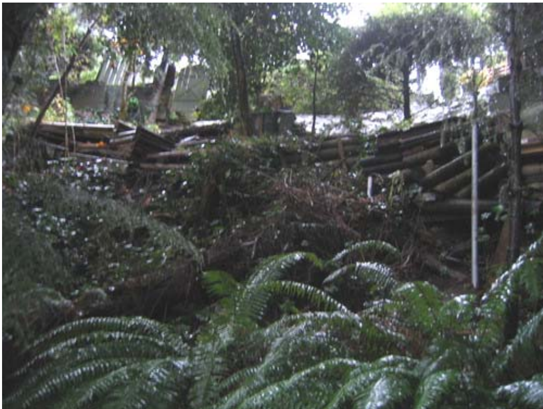
Figure 2. 1305 Lennox Street – View up-slope at timber crib wall
