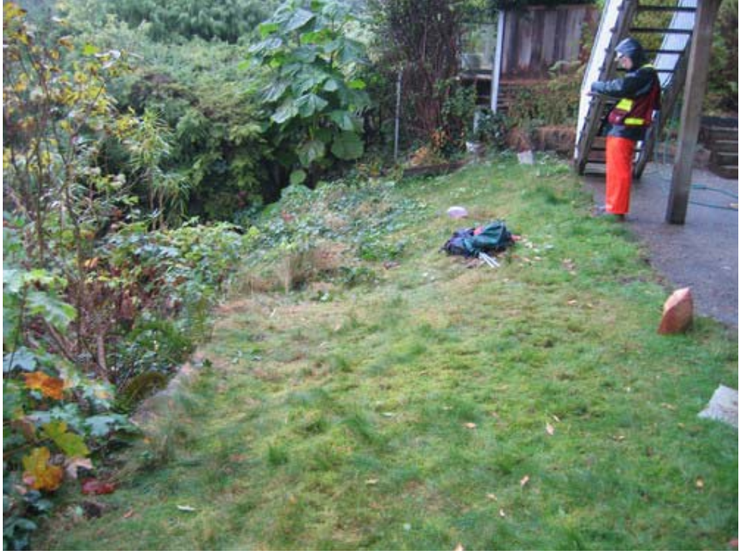
Figure 3. 1279 Lennox Street – View looking north at slumping backyard
