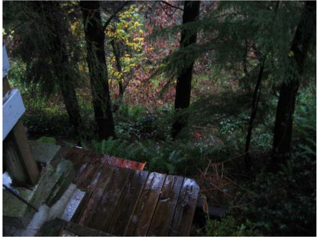
Figure 4. 1305 Lennox Street – View down-slope from just below the crest
