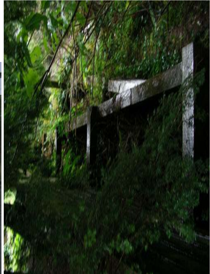
Figure 2. 1345 Lennox Street – View looking NW along timber crib retaining wall
