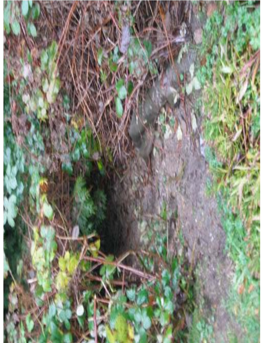
Figure 4. 1425 Lennox Street – Exit of drainage at slope crest
