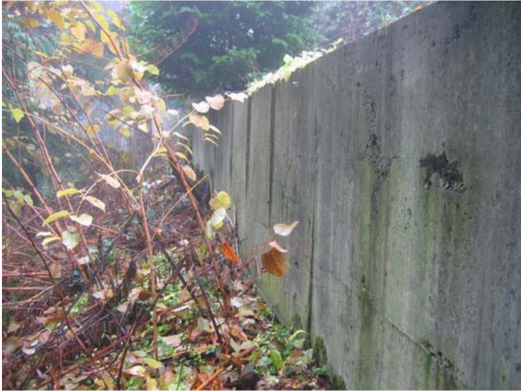
Figure 3. 1491 Lennox Street – Concrete retaining wall (lower wall)
