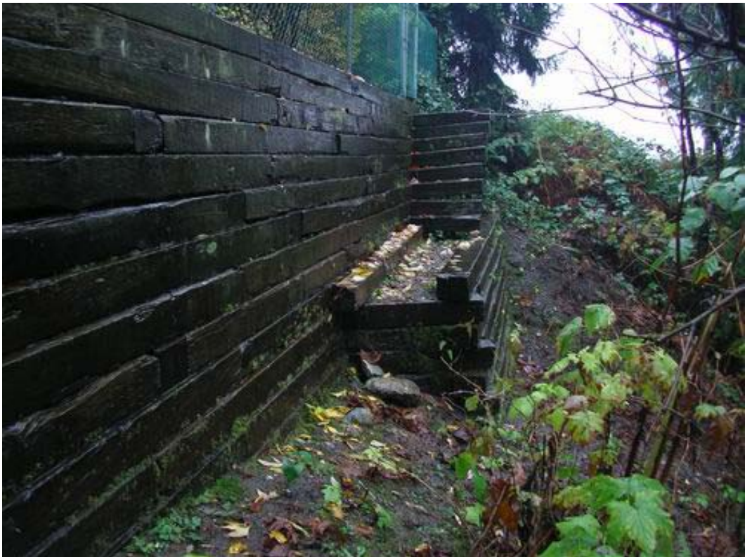
Figure 4. 1477 Lennox Street – Timber crib retaining wall
