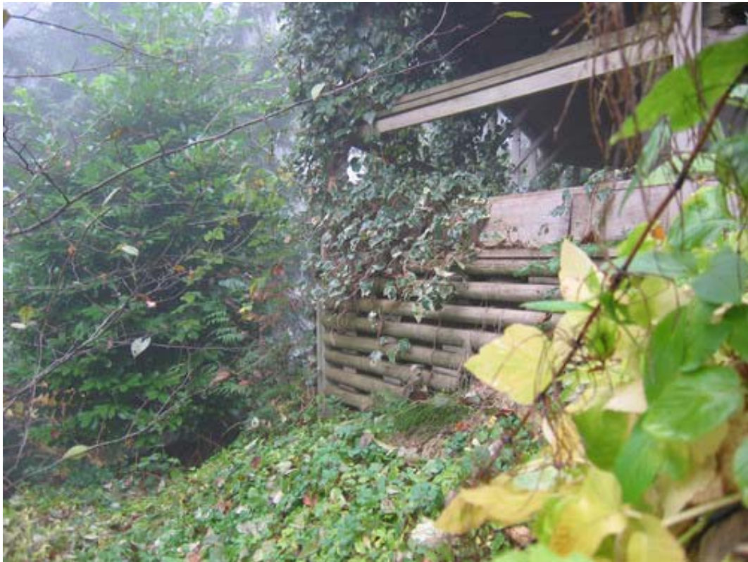
Figure 4. 1491 Lennox Street – Deck and timber crib retaining wall (upper wall)
