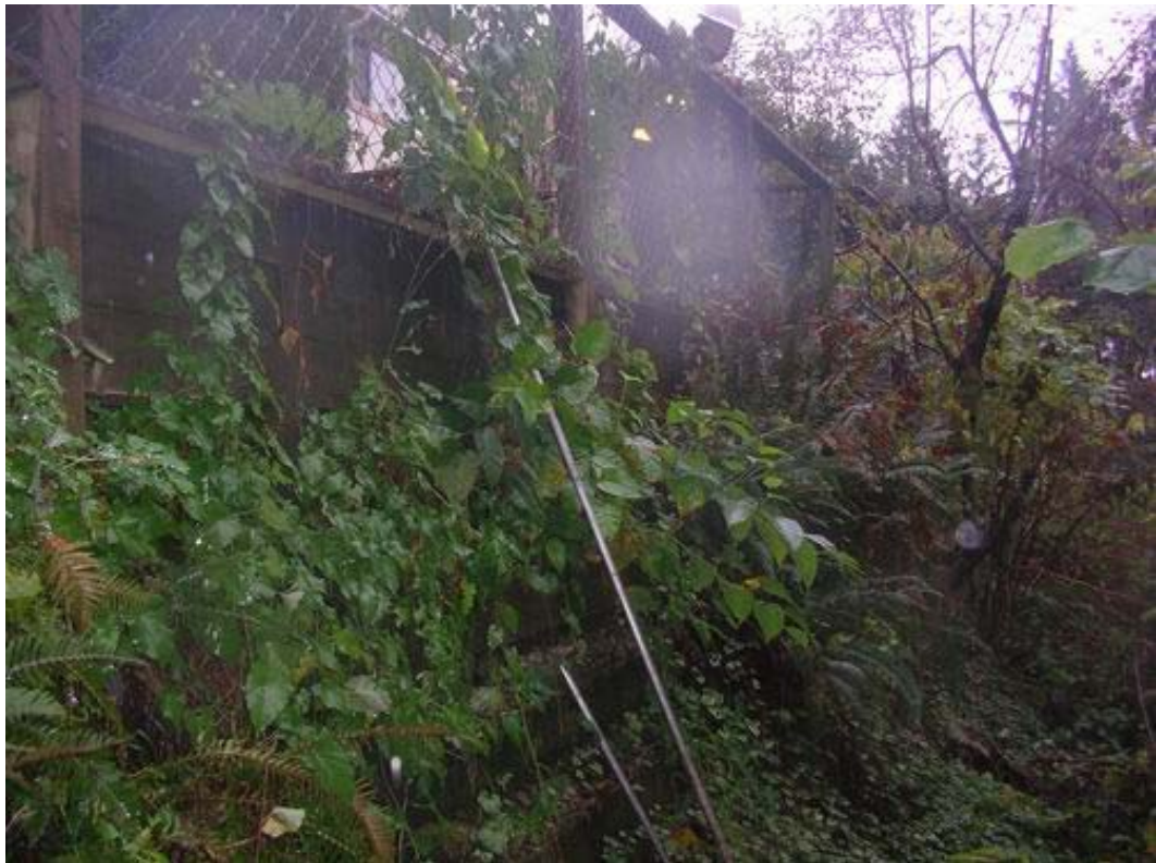
Figure 4. 1479 Lennox Street – Timber crib retaining wall
