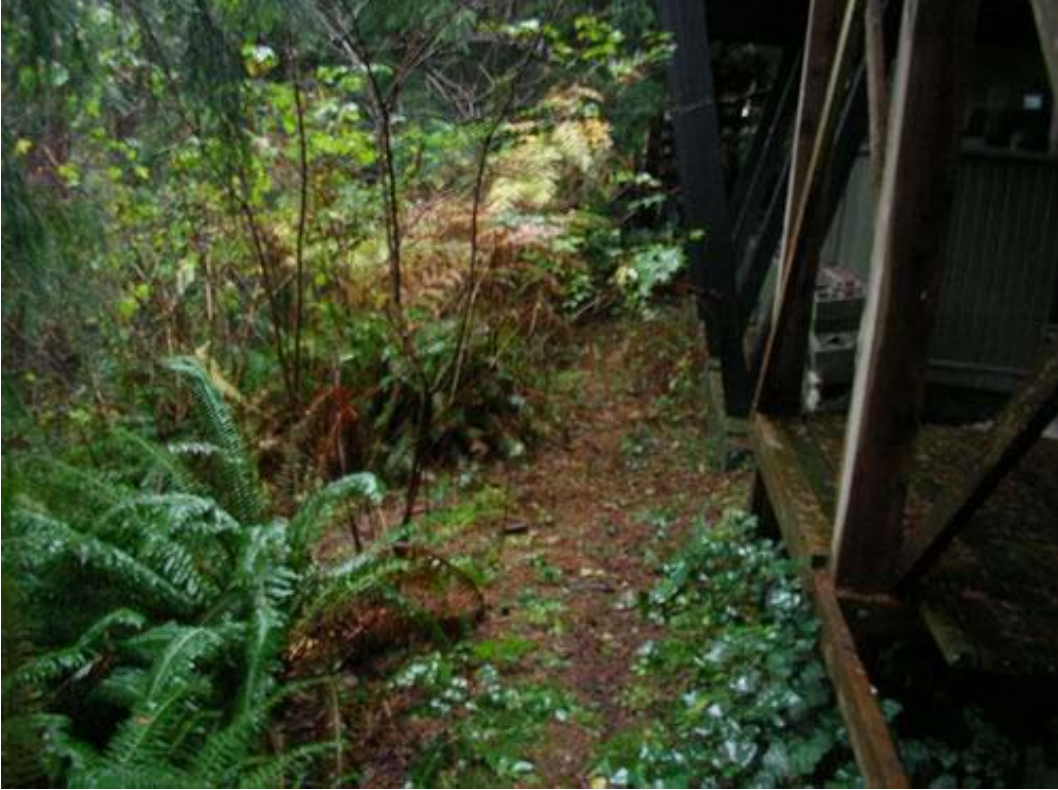
Figure 3. 1583 Lennox Street - View of slope crest looking north
