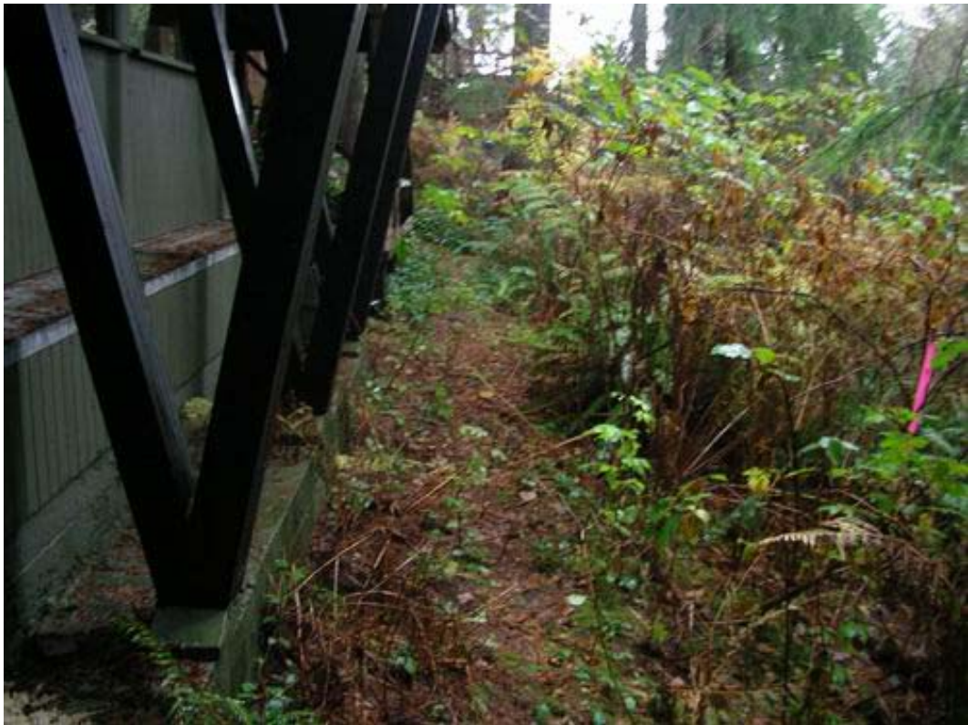
Figure 2. 1583 Lennox Street – View of slope crest looking south
