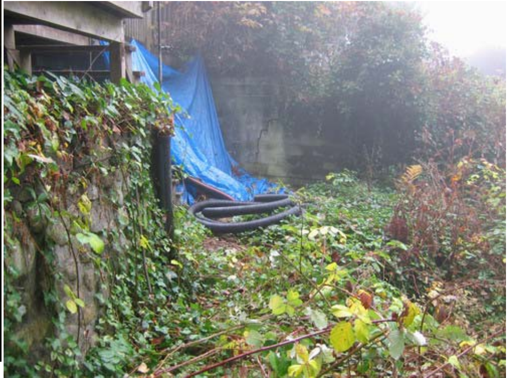
Figure 4. 1557 Lennox Street – View looking south along crest
