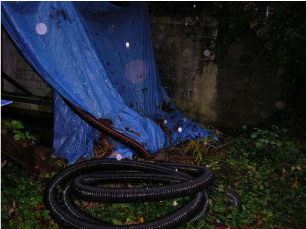
Figure 2. 1557 Lennox Street – Drainage pipe exiting house, draining downslope
