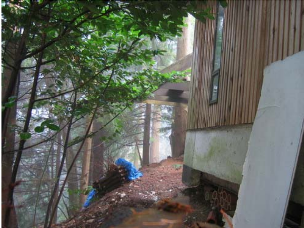
Figure 3. 2414 Swinburne Avenue – View north along fenceline (backyard)
