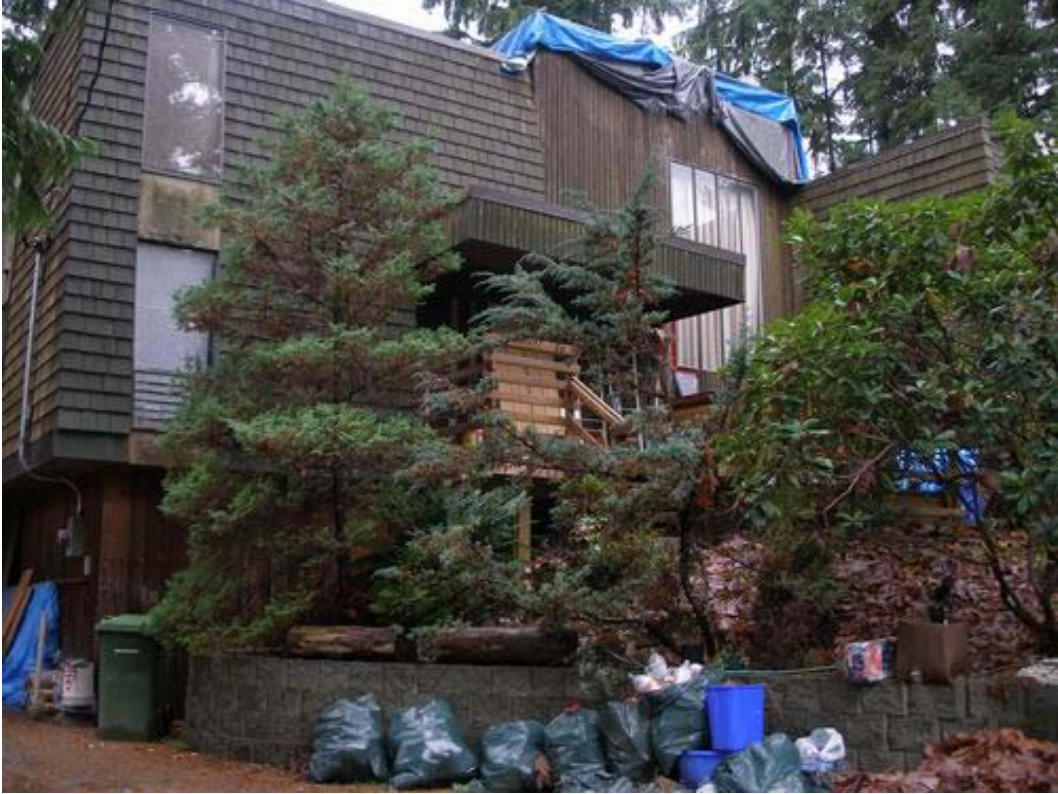
Figure 1. 2414 Swinburne Avenue – Front of the house
