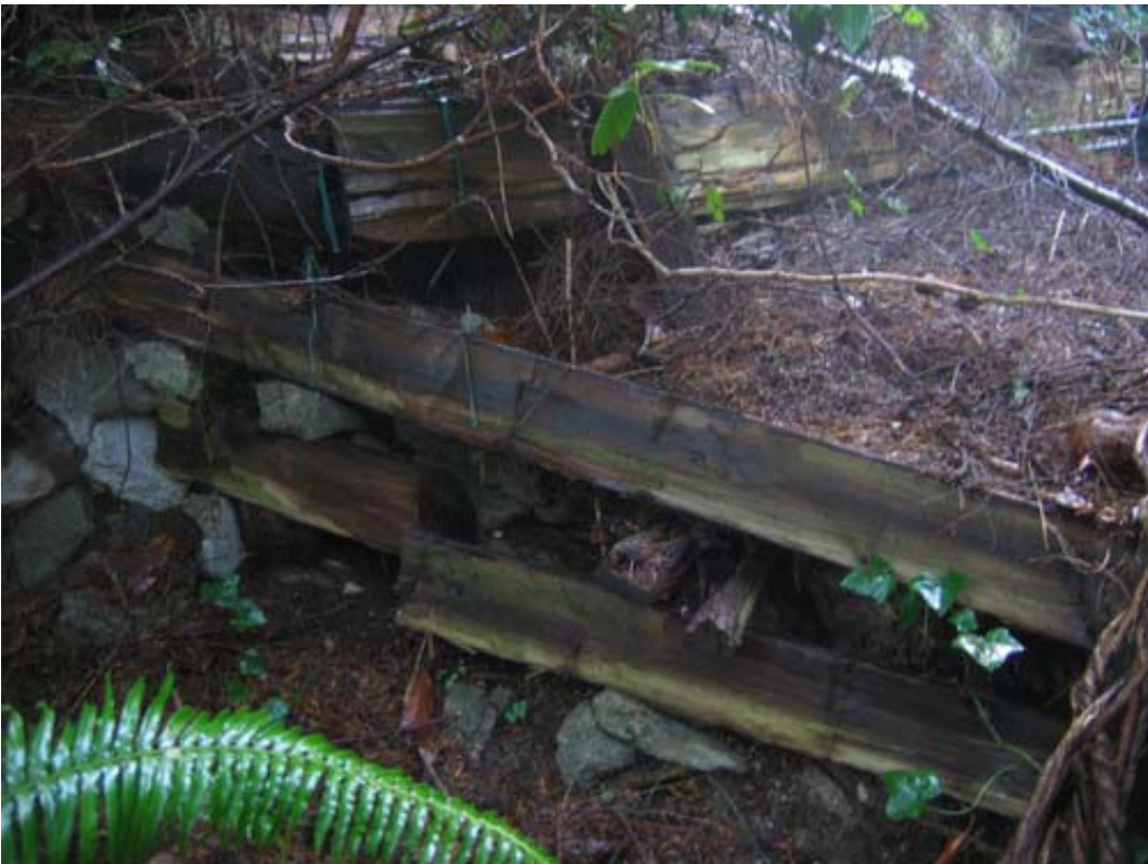
Figure 2. 2402 Swinburne Avenue – Retaining wall
