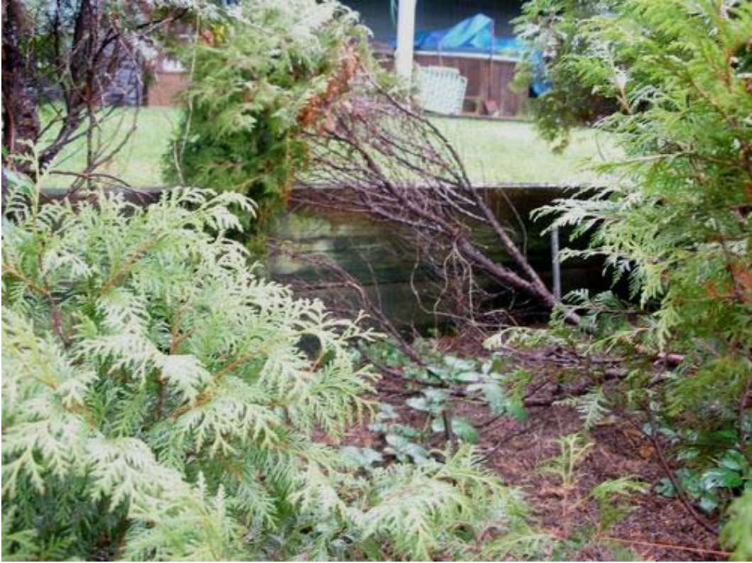
Figure 3. 1775 Layton Drive – Timber retaining wall
